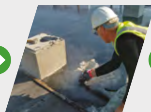
Easily worked with a float or squeegee
