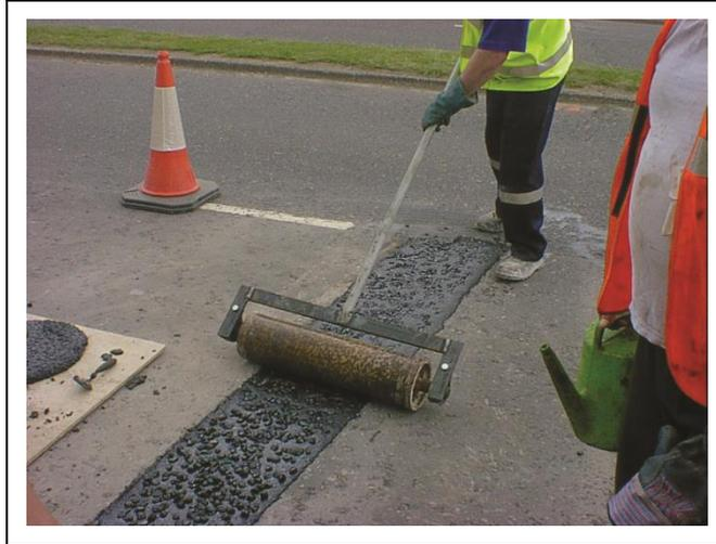
12.8 Before opening to traffic the installer must conduct a visual check for uneven surface texture and any other discernible faults, and carry out remedial work if necessary.
