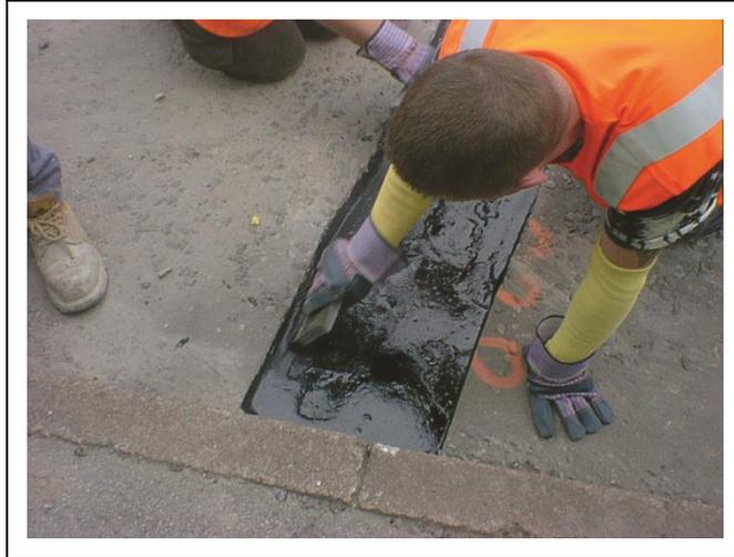
12.4 Permatrack H blocks do not contain the required amount of coarse aggregate which is added during the re-melt process. The blocks are broken into suitably sized pieces and melted in a mechanically agitated mixer. The coarse aggregate is supplied in pre-weighed 25 kg bags and the required amount is added to the mixer. The two components are thoroughly mixed together until homogeneous. The ratio of Permatrack H block to coarse aggregate is 65 : 35 by weight.
