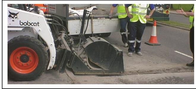
11.2 The recessed area and local road surface are swept, spoil is removed, and the recess is dried and cleaned using hot compressed air (see Figure 2).
