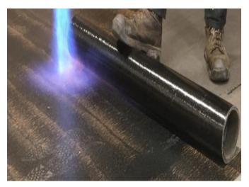
Figure 3 - Typical torch on method of application
