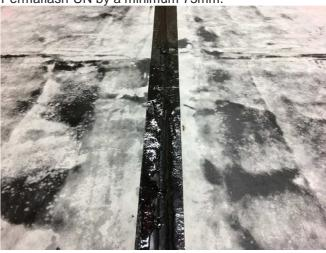
Detail is completed by the installation of the Permaguard-F protection sheet bonded into the final coat of Permatec
