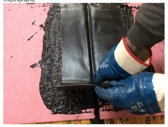
Permaflash-UN must be installed with minimum 150mm end laps fully bonded and sealed in hot Permatec compound.
