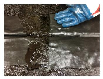
The installed IKO Permaflash-UN must not be left exposed to damage and must be fully protected by the installation of the full Permatec system without un-due delay.
