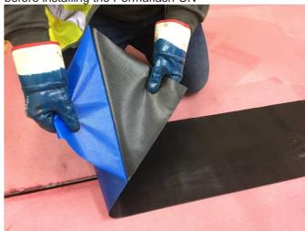
Permaflash-UN is fully bonded in hot Permatec compound centrally over the movement joint. Care being taken to ensure that an excess of Permatec extrudes beyond the edges of the Permaflash-UN.
