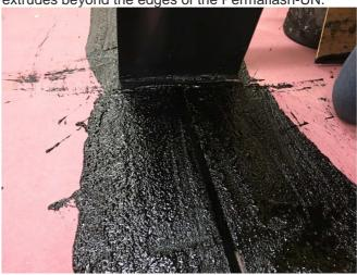
Ensure Permaflash-UN is pressed into the expansion joint gap to form a minimum 10mm loop in the membrane
