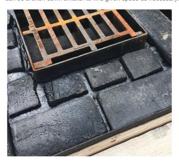
9.5. Once the IKO Pacopatch Bricks are in position, the grout should be allowed to cool for at least 10 mins before flooding the rebate with molten IKO Pacopatch Grout, filing all the voids around the IKO Pacopatch Bricks. A further layer of IKO Pacopatch Grout is then installed up to 20mm below road level. Allow to cool for a further 10 mins.
