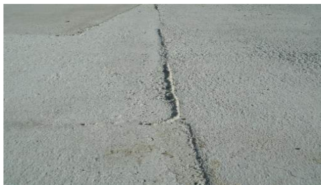
Typical raised float ridge
