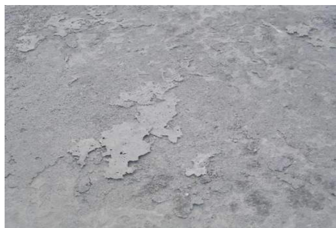
Example of surface laitance
