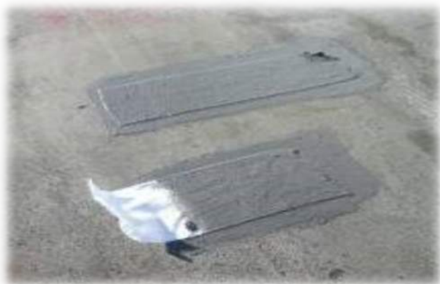
Embed a strip of polyester fabric into the roof coating and allow to cure completely
