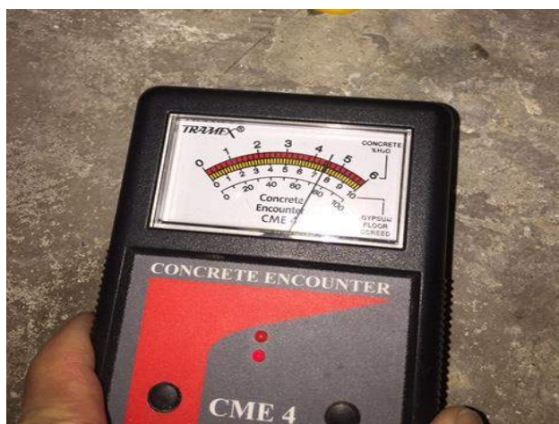
Moisture content reading should be within 6%
