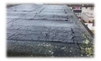
Core sampling of the roof build up in several different locations should then be used to establish the full build up and history of the roof. If documentation is unavailable, and/or an internal inspection is impractical, such core sampling is essential.
