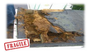
All decks where wood particle board or chip board is found these must be removed and replaced with a non-fragile alternative.
