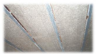
Using pertinent safety measures, an external inspection should follow, which may reveal deflections due to collapse between joists, or other deck damage.
