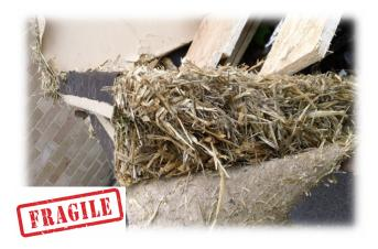
Strammit decks were used as a roof deck material from the mid-1950s. However due to the long term structural stability, especially if contaminated by moisture is now regarded as a fragile material under the guidance in HSG33 from the Health and Safety Executive.
