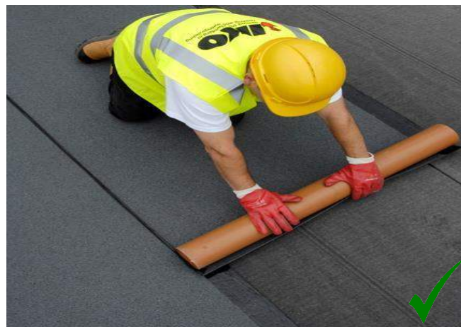
IKO Ultra H-A underlay with weighted roll bar.
