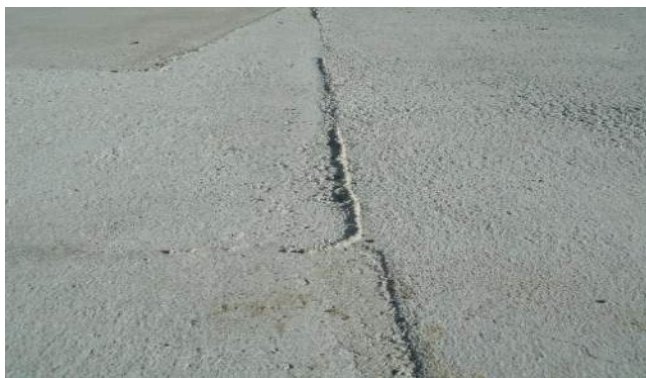
Typical raised float ridge
