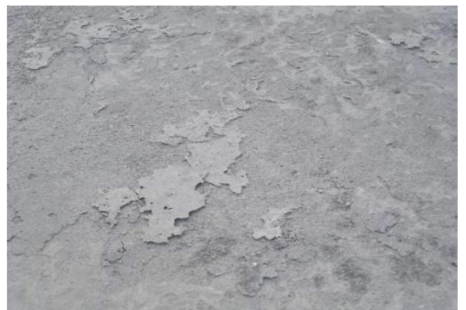
Example of surface laitance
