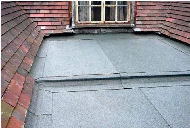
Pitched roof abutments
