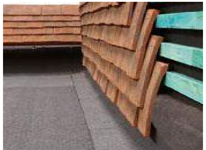
Vertical hanging tiles
