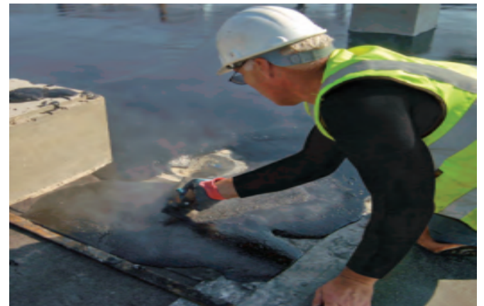
Typical application of a mastic asphalt screed application
