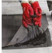
Allow the IKO Permamatec to cool completely before checking the bond strength. The bond to the substrate is checked by folding back the loose edge(s) of IKO Permagaard-F and pulling it towards you.
