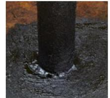
Exposed pipe flashings must be protected with IKO Permaguard-M Protection Sheet, which is applied by controlled torch application and the upper edge protected with a cover flashing to complete the detailing.
