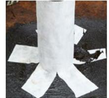
The height of the IKO Permateg System should be at least 150mm above the finished roof level.
