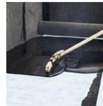
Ensure that the IKO Permateg membrane is taken beyond the width of the IKO Permaguard-F protection sheet on both edges, which is also 1m wide.
