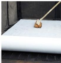
Once one row of the IKO Permateg membrane and fabric has been applied, another row can be started. The membrane should overlap the fabric from the preceding row by approximately 100mm, enabling the next roll of IKO Permaflash-R to be embedded into the membrane to form a minimum, fully-bonded 75mm overlap between the two sheets of fabric.
