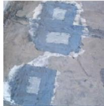
Where possible, the protection layer should first be carefully removed, exposing not only the damaged membrane, but also at least 75mm in all directions from it. If the protection layer cannot be removed without causing further damage to the underlying IKO Permateg, the upper surface should be carefully heated with a gas torch to 'sweat' the bitumen within it.
