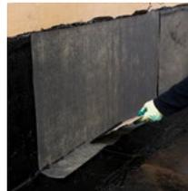
Laps in IKO Permaguard-F protection are to be minimum 75mm and fully sealed using hot IKO Permateg.
