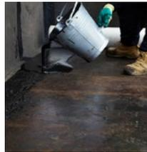
Using the squeegee, pull the hot IKO Permaterc compound towards you in a methodical manner, ensuring that it covers the substrate beyond the width of the IKO Permaflash-R Reinforcement, which is 1m wide.
