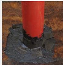
Two coats of IKO Permateg, incorporating IKO Permaflash-R, are applied to the pipe.
