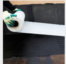
As the IKO Permaflash-R is being installed, it should be brushed into the hot IKO Permateg, taking care to avoid air pockets, folds or wrinkles in the fabric.
