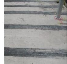
Where a structural topping is not required, IKO Permateg can be applied directly to the pre-cast concrete units, providing they are finished to a suitable quality. The surface will need to be the equivalent of a skip float or power float finish, and the units installed sufficiently level and even to ensure roof drainage is not adversely impacted.
