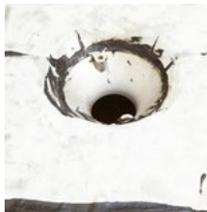
The second coat of IKO Permasec is applied as soon as possible and must fully cover the IKO Permaflash-R reinforcement. Spread evenly, the second coat is also applied at a nominal thickness of 3mm.
