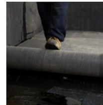
With subsequent rows, ensure that the second coat of IKO Permateg overlaps on to the preceding row by approximately 100mm, enabling a minimum 75mm sealed lap to be formed.
