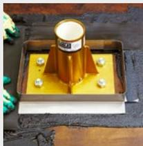
The former is then filled flush with hot IKO Permaterc. Depending on the size, several pours may be required, leaving the IKO Permaterc to cool each time.
