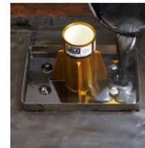
Once filled, IKO Permaguard-F should be applied to the top and sides of the pitch pocket and bonded to the surrounding flat to complete the detail.
