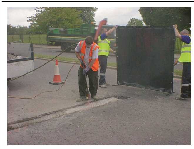
Figure 2 Drying using hot compressed air
