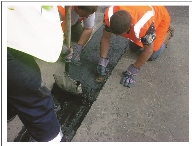
Figure 4 Application of Permatrack H
