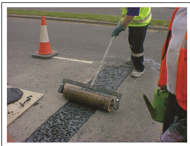
Figure 5 Rolling in pre-coated chippings
