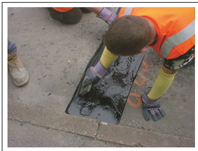
Figure 3 Application of Permatrack PSB to recess
