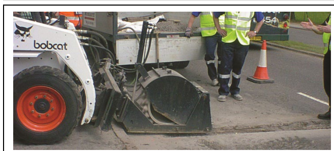
Figure 1 Mechanical planing out of cracks
